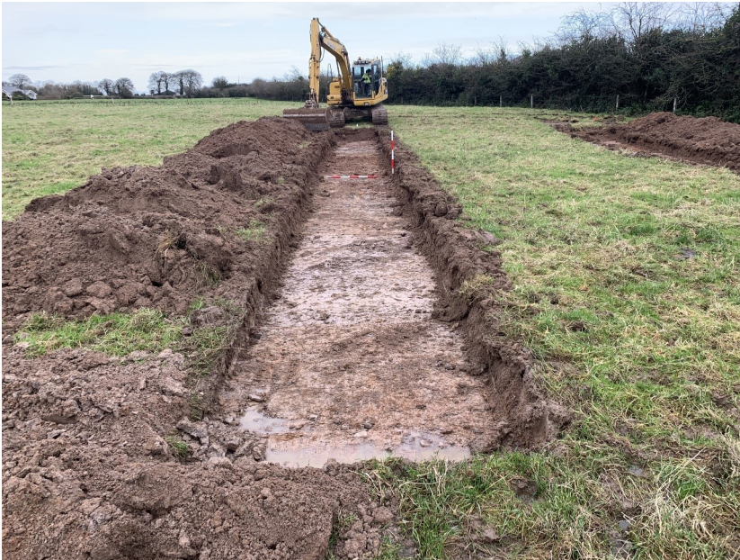
Plate 19: Test Trench 7, facing northeast
