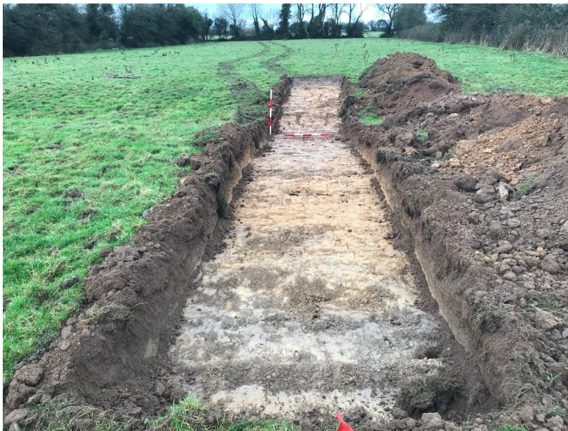
Plate 23: Test Trench 10, facing north
